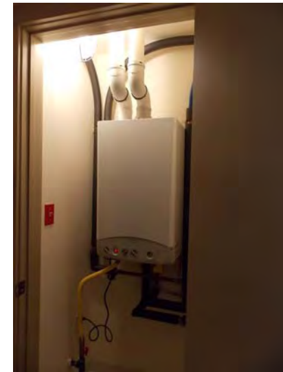
Each apartment has been upgraded with its own on-demand gas-fired boiler, which produces hydronic heat and DHW.
