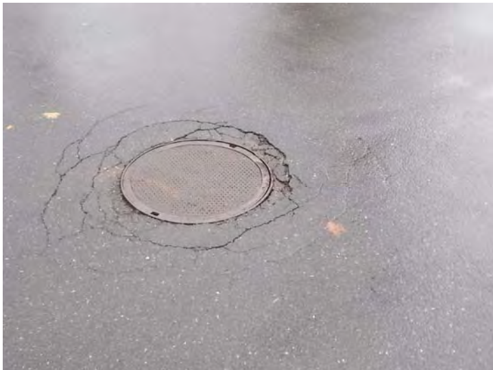
A close-up of surface cracks around a manhole cover.
