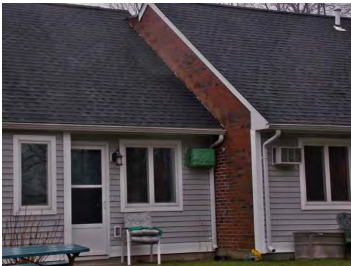
Residential buildings have mostly vinyl siding with bricked parting walls.
