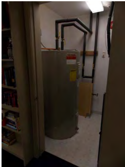
An electric heated DHW tank that serves the community building.
