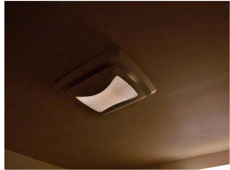
Apartment bathrooms feature new ceiling fan/light fixtures. Fans are variable speed, responding to varying moisture levels.
