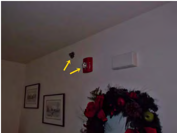
A fire sprinkler head and a horn/strobe in an apartment.
