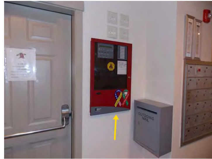
The central fire alarm control panel (FACP) is located in the community building.
