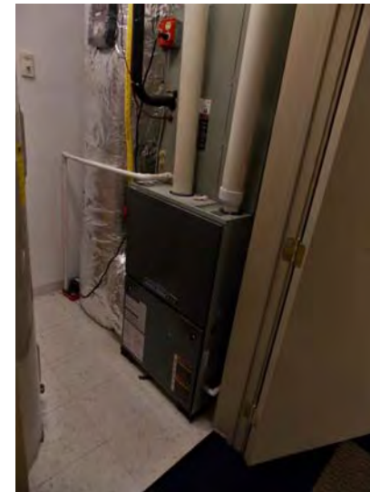
This is one of the condensing furnaces that serves the community building.
