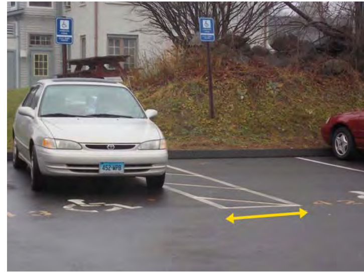
The access aisle at this designated parking space should be re-striped to a width of five feet.
