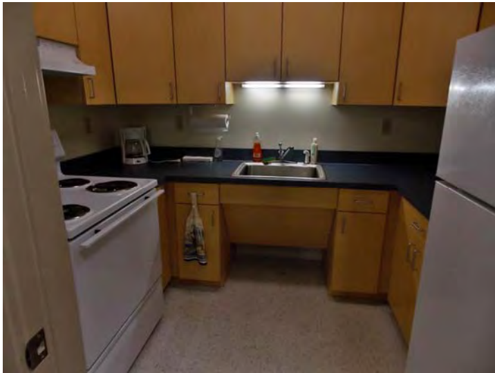
The community kitchen should be updated to include a 30-inch work surface with adequate knee space.
