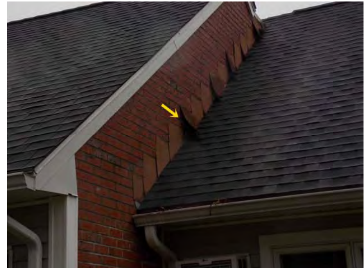
A close-up view of loose step flashing (rear of Building D).
